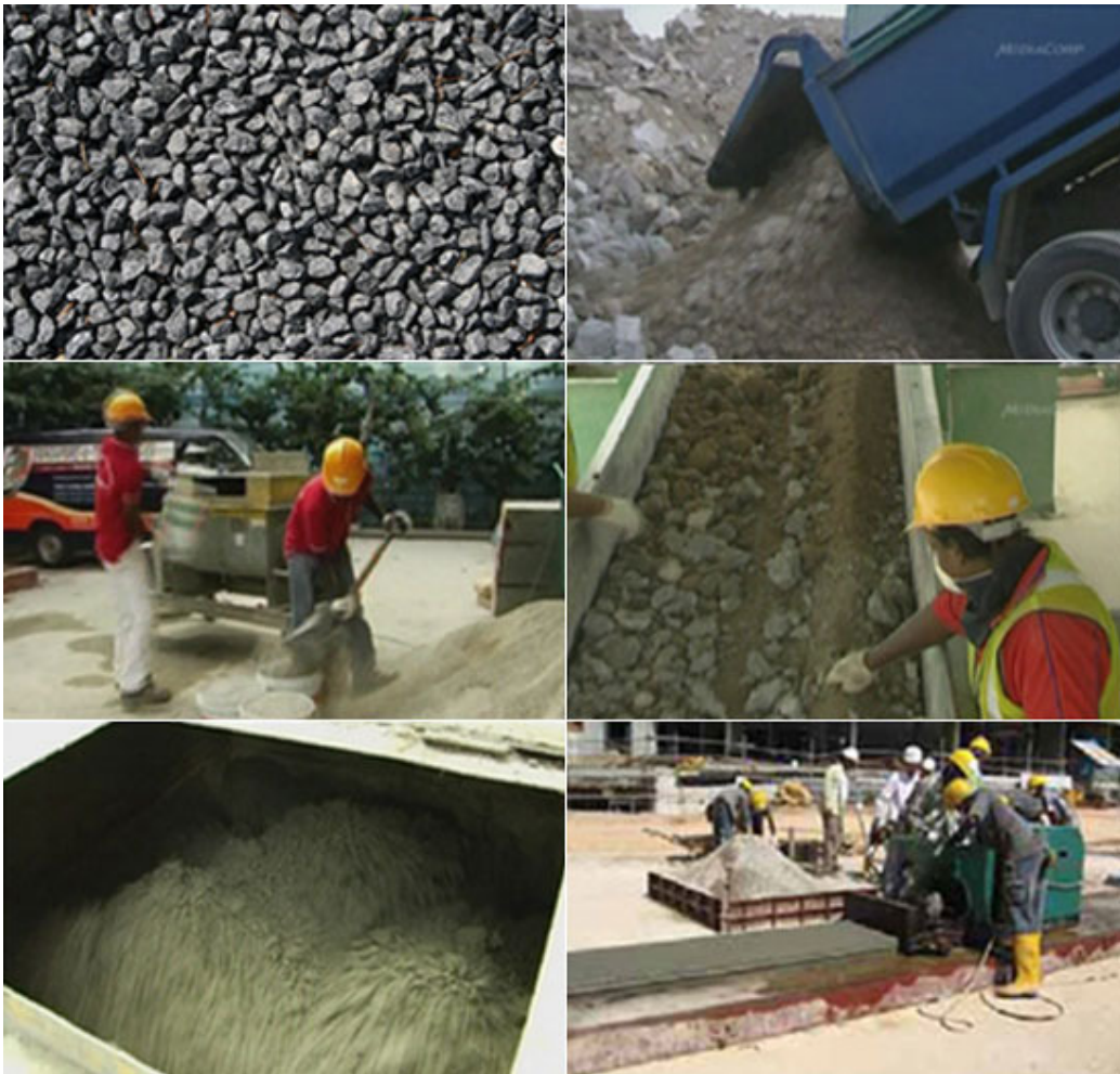
process of concrete re-use in situ
